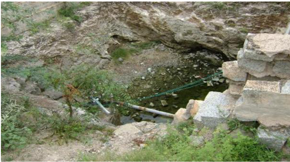
Over Exploitation of Groundwater: Existence of Inwell Bores
