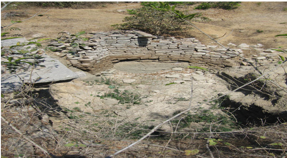
Over Exploitation of Groundwater: Failure of Dugwells
